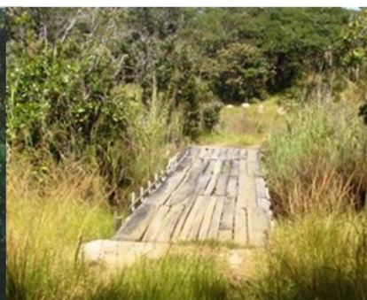
Thick Euc. planks on a bus frame
